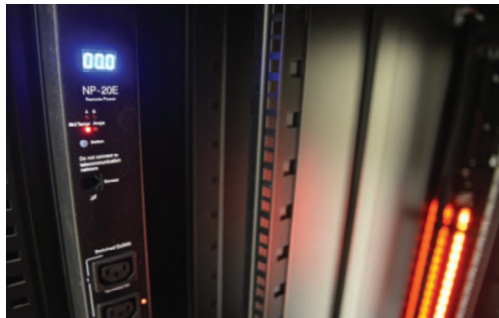
Smart network enabled PDU
