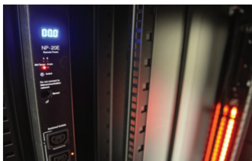
Smart network enabled PDU
